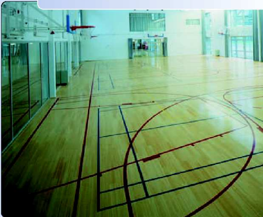
Fixed permanent installation, bamboo flooring
